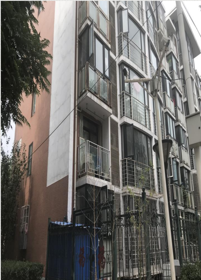
Source: Spruce Point private investigators
